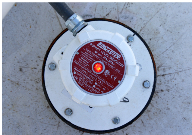
Point level sensors alert to full status to prevent overfilling silos.
