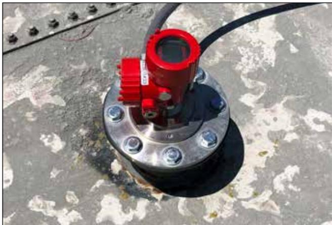
ResinView is compatible with many types of level sensors. Granular, powder, flake, or liquid forms of resin may require different types of sensor technology. Non-contact radars, SmartBobs, and lasers are often used for resin monitoring. No power to the bin, no problem—battery powered sensors make installation easy. ResinView™ SaaS is compatible with sensors using analog or 4-20 mA, Modbus, or HART outputs.
