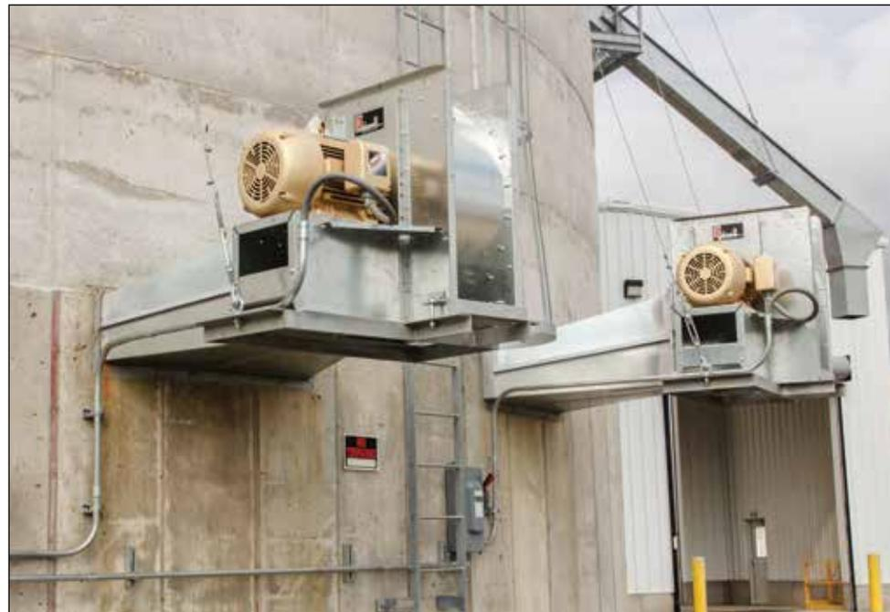
Two of four Caldwell 40-hp centrifugal aeration fans that deliver roughly 1/10 cfm per bushel to stored grain. Ground picture courtesy of EBM Construction.
