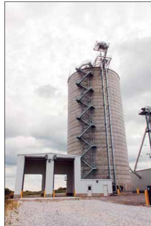
Ground-level view of the new annex with twin enclosed receiving pits, Hoffmann 350,000-bushel concrete storage silo with Warrior switchback staircase, and free-standing Schlegel 20,000-bph leg.
