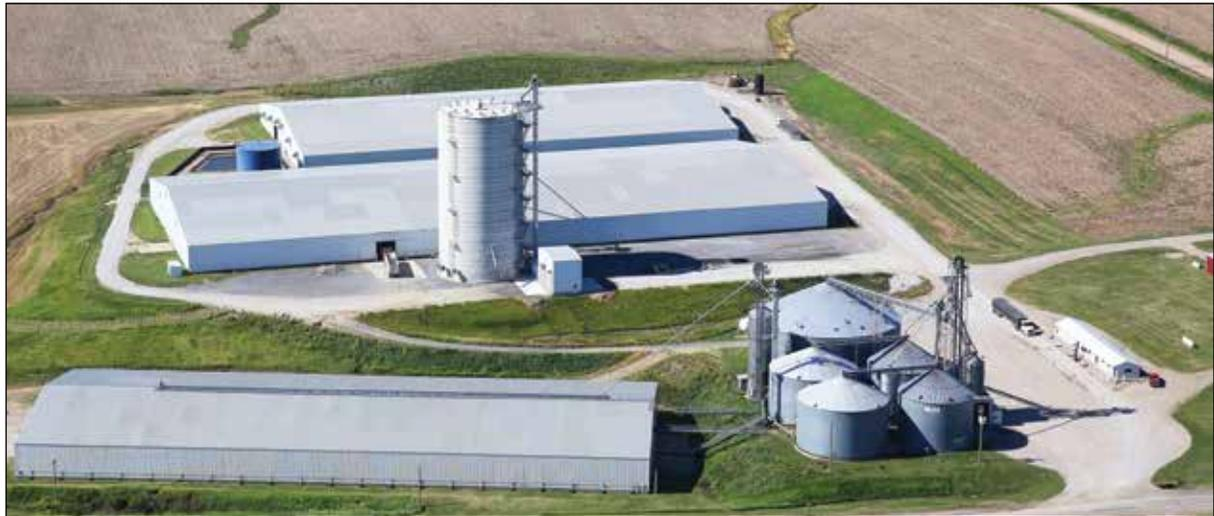
*Cooperative Supply Inc.'s grain elevator at Dodge, NE, with new jumpform concrete storage silo and freestanding leg adjacent to a 2-million-bushel soybean flat storage. Aerial photo courtesy of Dakota Aerials, Yankton, SD.*
