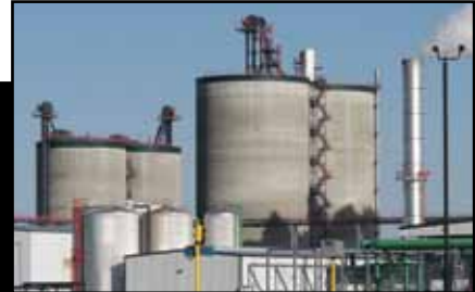
Nebraska Ethanol Plant
