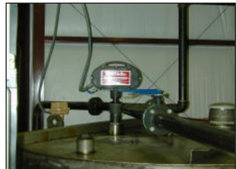
**SmartBob II remote measuring mineral oil on an indoor liquid tank**
