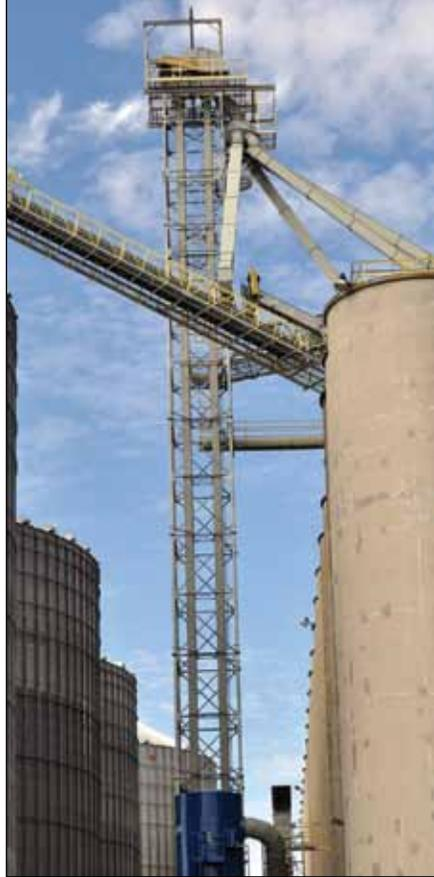
*Twin receiving pits and 30,000-bph Hawthorne-Seving receiving leg, which feeds into a six-hole Hayes & Stolz distributor. Photo by Ed Zdrojewski.*
