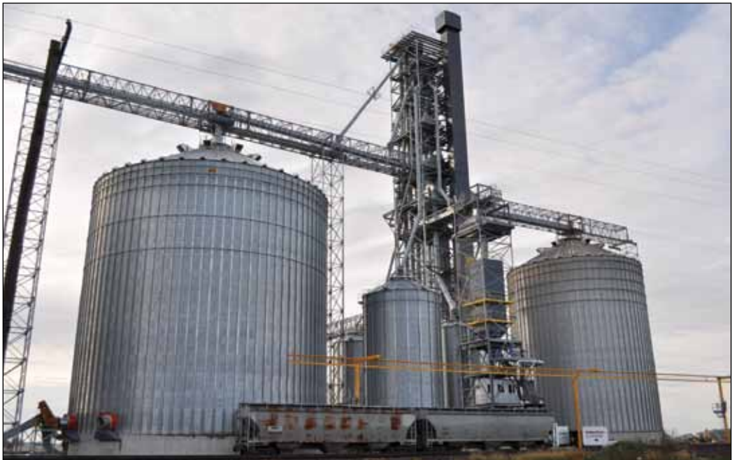
Closeup view of the newest construction at the Milmine elevator, including five corrugated steel tanks, four legs, a tower dryer, and bulk weigh loadout system for origin weights. Ground level photos by Ed Zdrojewski.
