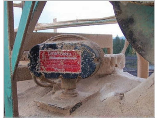
SmartBob installed on a sawdust bin.
